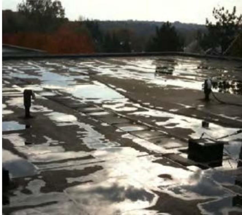
There are roof drains, but the roof is flat and uneven and water does pool in many spots after rains. A puncture in one of these areas could cause a lot of water damage, and moisture problems like mold, inside the building.
