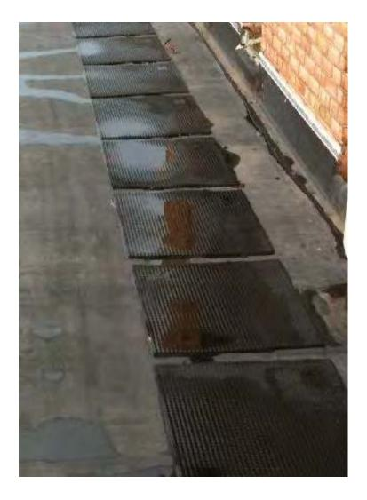
Likely roof travel paths have traction mats bonded in place that protect the membrane.
