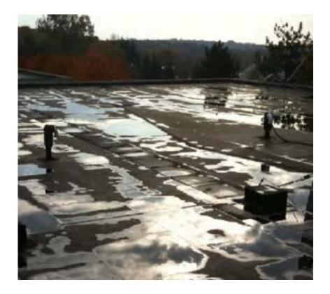
There are roof drains, but the roof is flat and uneven and water does pool in many spots after rains. A puncture in one of these areas could cause a lot of water damage, and moisture problems like mold, inside the building. • There is a large raised metal platform that should be used for roof activities unless the equipment or experiment requires otherwise
